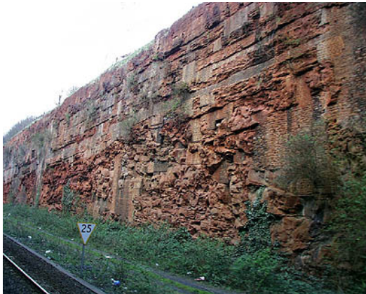
St Annes' railway cutting
