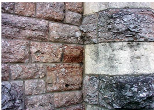
The Joint Station of the 1800s is made of squared, coursed rough Dolomitic Conglomerate blocks, contrasting with smooth Bath Stone ashlar. The Triassic conglomerate consists of rounded pebbles of grey Carboniferous Limestone in a reddish fine matrix that contains the minerals hæmatite and dolomite. It came from quarries at Draycott, near Cheddar, on the other side of the Mendip Hills. Recent repairs were done by excavating similar stone from a small old quarry in
