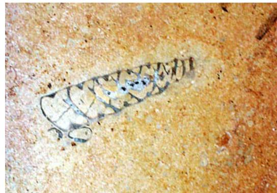
You will need a ticket for the next stone. Machine-cut slabs of limestone from France were used for paving part of platform 3 in 2000. It is Rocheret Jaune, an Early Cretaceous limestone that comes from Belley, near Lyon. Beautiful sections through fossil shells, especially high-spired gastropods, can be seen in places. The same stone has been used for paving at Paddington Station and at both ends of the Channel Tunnel, as well as in Bristol's Centre and Millennium Square.
